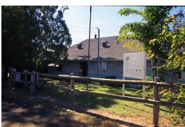
Pine Creek Repeater Station
