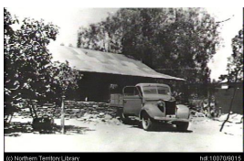
Griffiths House - building new boys dormitory
