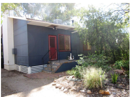
Exterior of house in Warburton Street, Alice Springs
