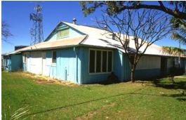
Pine Creek Repeater Station
