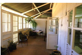
Pine Creek Repeater Station
