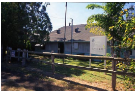
Pine Creek Repeater Station
