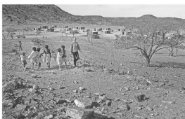
Aboriginal housing at Santa Teresa Mission south of Alice Springs, Northern Territory, 1966
