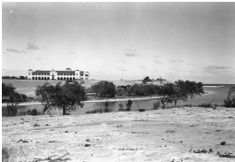
Nazareth House on the Chapman River, Geraldton, 1946
