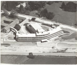
Mersey General Hospital from the air
