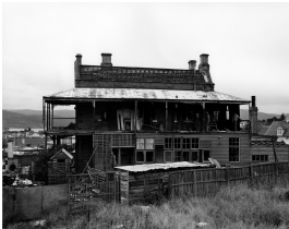
The Normal School, later the Hobart Town Female Refuge, and then the Anchorage Home - before demolition
