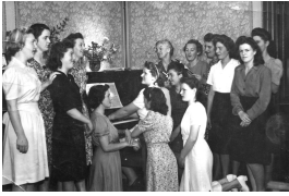
Women gathered around a piano at Tower House Young Women's Hostel
