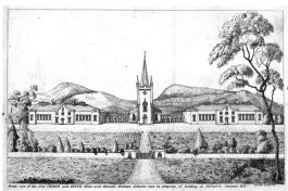
Front view of the New Church and King's Male and Female Orphan Schools now in progress of building at New Town, January 1831
