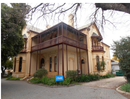
Former building entrance, Salvation Army Boys' Home, Kent Town
