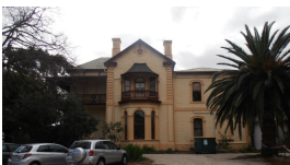
Side of former building, Salvation Army Boys' Home, Kent Town
