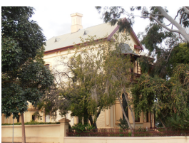
Former building, Salvation Army Boys' Home, Kent Town
