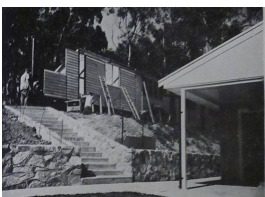
Woorabinda Campsite under construction
