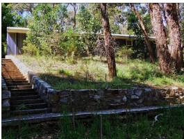
Former Hostel Building at Lake Woorabinda
