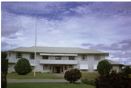
Main entrance, Mossman Hall Psychiatric Hospital, Charter Towers
