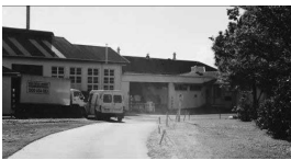
Holy Cross entry/despatch section of laundry building
