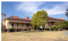
Original buildings, Riverview
