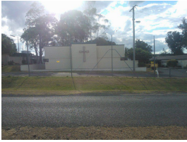
Chapel, Darling Downs Correctional Centre
