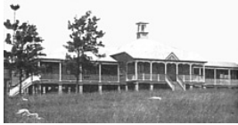
Rockhampton Receiving Depot c.1913
