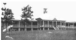
Rockhampton Receiving Depot c.1913
