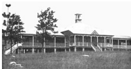
Rockhampton Receiving Depot c.1913
