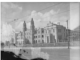
Deaf, Dumb and Blind Institute building, Darlington
