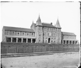
Deaf, Dumb & Blind Institute, before extensive renovation and addition, Sydney
