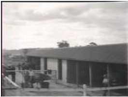
The dairy and stables, Brush Farm
