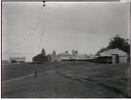
Brush Farm Reformatory quarters
