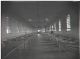
Brush Farm Reformatory dormitory
