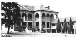
Eastern side of St Michael's Orphanage Baulkham Hills 1940s
