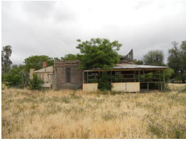
The northern side of the former girls' dormitory [former Warangesda Station]
