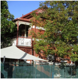
Former Salvation Army Creche at 481 Canning Street, North Carlton
