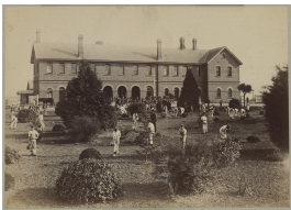
Boys' Reformatory, Ballarat
