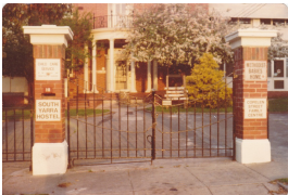
Front gates at 12 Copelen Street, South Yarra
