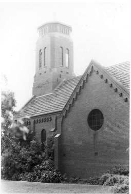
Phillip Island. Newhaven. St. Paul's Discovery Centre [chapel exterior]
