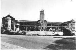
St Augustine's Building
