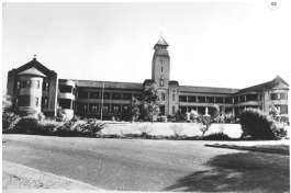
St Augustine's Building
