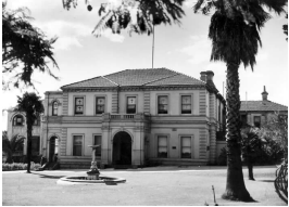
St Anthony's Home, Kew, building
